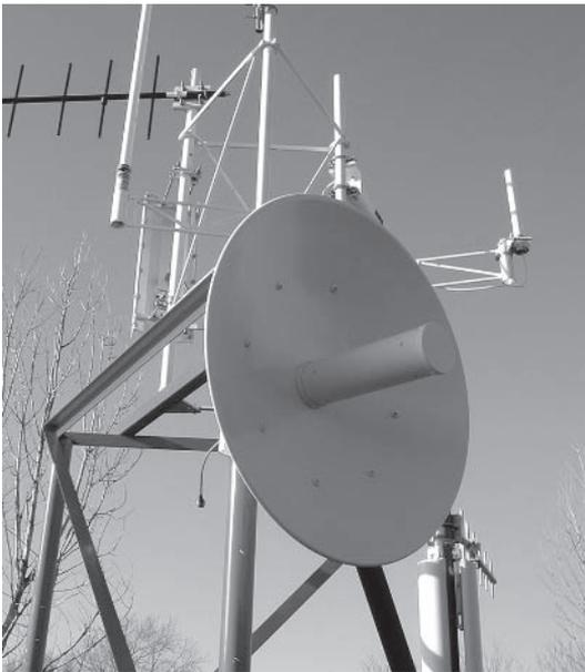
**Figure 2-8a: Dish Antenna.** Photo(s) and illustration(s) reprinted with the permission of MAXRAD, Inc.
